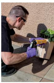
Apply the adhesive on a clean substrate in vertical beads or dots.
