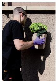
Use sufficient hand pressure to ensure good wetting on rough substrates.
