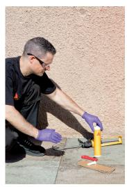
Mount the V-cut nozzle and insert the cartridge into the gun.
