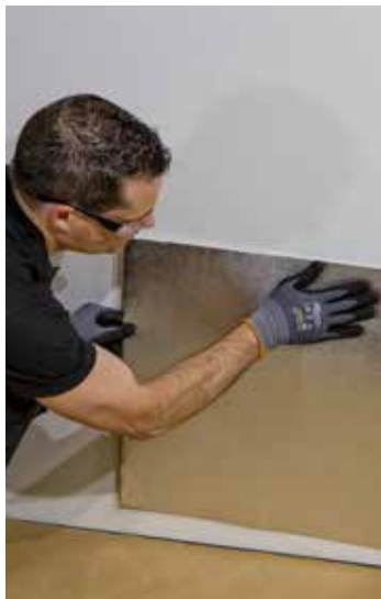
Installation and assembly works.
