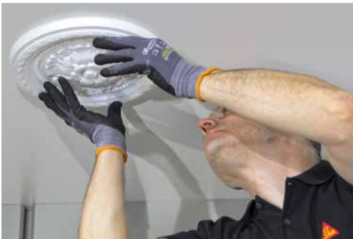
Interior decoration works.
